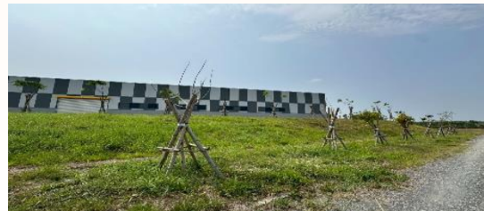
Greenery around the construction
